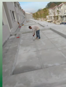
Apply TMS 600 at Grooveline of Concrete Rooftop TMS-600 屋顶水泥面伸缩缝施工
