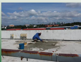
Teson Slurry Flex TW-151 Crack Line Repair
