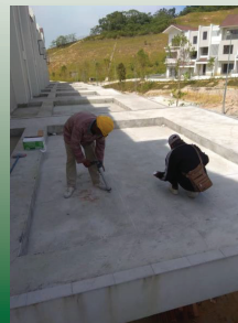
Apply TMS 600 at Grooveline of Concrete Rooftop TMS-600 屋顶水泥面伸缩缝施工
